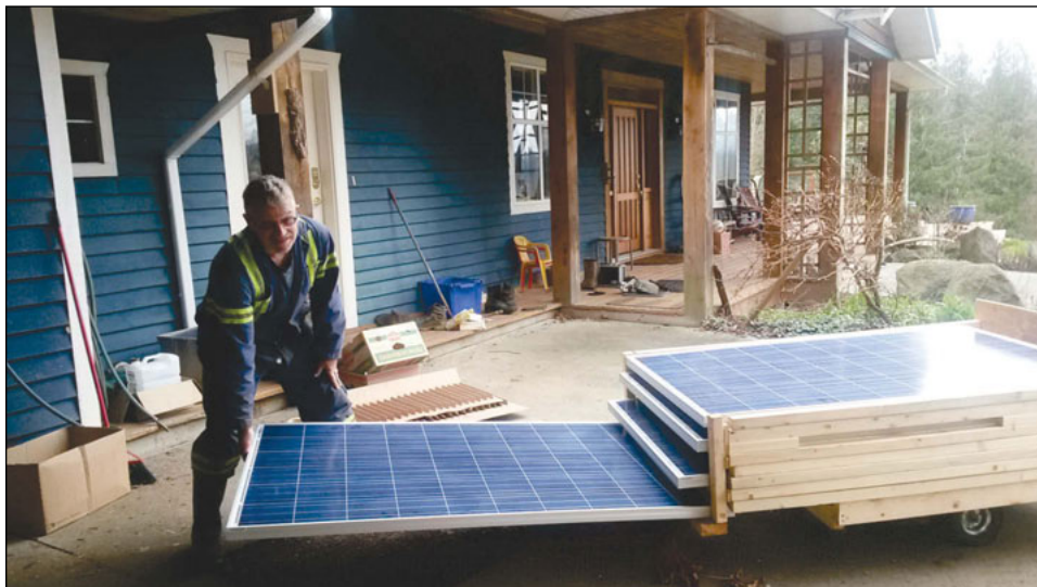
A cart was made for transporting the panels to the yard.
