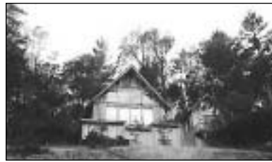
De Courcy Island: 152 ft of oceanfront, all season cottage, large deck with hot tub, 2 woodstoves, 4000w generator, deep well, lovely oceanviews. $269,000
